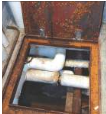
A hatch used to gain access to the pipes and steam tunnels at WUHS/MS. The hatch is only about 18 inches square, so in order to get replacement pipes through it, the pipes would either need to be cut into tiny pieces or larger holes would need to be drilled through the floor. The hatch door also shows signs of rusting due to leaking steam, which has occurred at various points throughout the building. Robert Shumskis Photo
