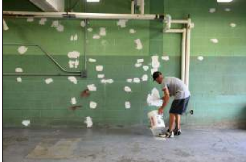
Dylon McCutcheon, who is part of the custodial and maintenance staff, works to turn what used to be a wood shop into a virtual reality classroom at Woodstock Union High School on last week in Woodstock.
